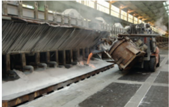
Kurri Kurri produces primary aluminium completed an upgrade in all operational areas during 2006.
