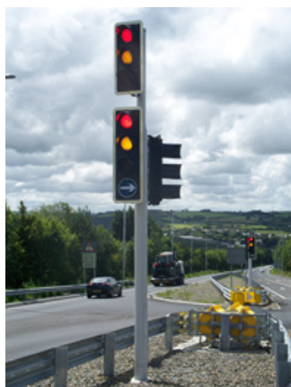
Traffic signal pole - Punch 165/145
