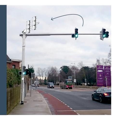
Rotating TRIs enable safe operations. Maintaining traffic signals on busy, multi lane carriageways is a costly, disruptive and potentially dangerous operation. A rotating mast arm can improve the safety of operatives whilst minimizing disruption to the travelling public.
