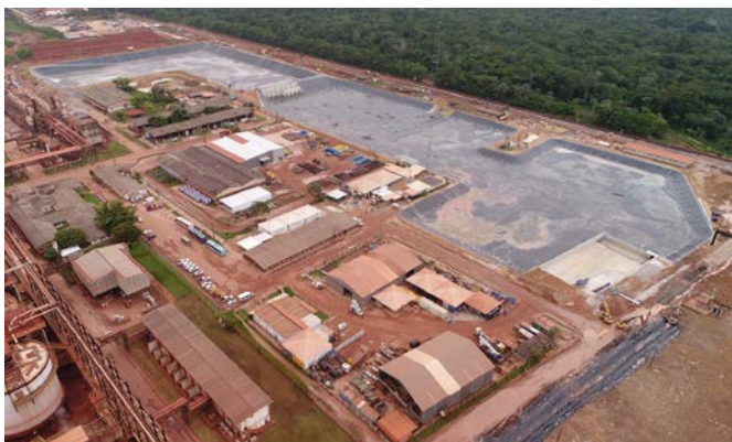
The water reservoir capacity at Alunorte has been increased by 350 percent since the rainfall event.
