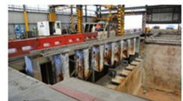
Removal of Crossover Duct and Support
