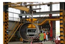
Removal of Crossover Duct and Support
