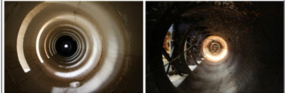
Both crossover ducts are now de-lined.
