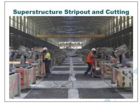
The next slide is lancing in half so that can be removed by forklift to the scrap lay down area where they then are further processed and cut up for recycling. You would have noticed a lot of metal on the pad now. We're basically half way through.
