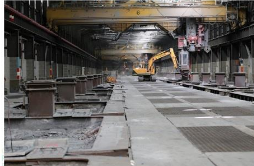
Pot Delining – Line 3 – Hammering 1st Cut SPL in April
