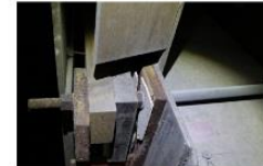
L2 busbar for KK175 pots - bonded ACM washers
