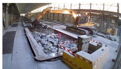
Pot Delining – Pulverising First Cut SPL – Trial in L2N
