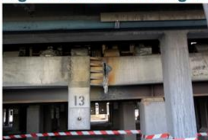
Line 1 cathode busbar after lancing. Note 100mm left at top and yawning gap. Will be removed by excavator during demolition.
