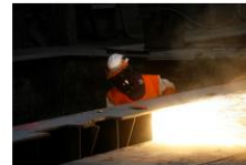
The pot shells weigh approximately 25 tonnes each. They are cut into five pieces of 5T each to make handling easier. Approximately 50mm of the deckplate is left uncut on both sides and will be broken up by a demolition excavator after the shell is pulled off its supports.
