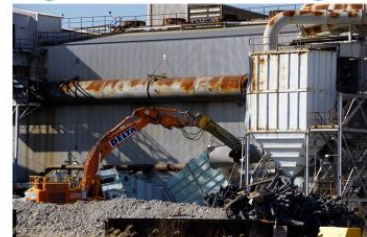
Demolition of Line 3 south dry scrubber baghouse.
