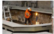
Oxy-propane cutting of pot shells in Line 1.
