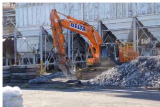
Pulverising of spare Potroom floor slabs - backfill for void filling.
