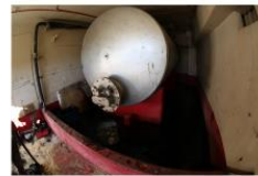
Heavy fuel oil tank in Casting. Fuel oil has leaked out but is contained within a bunded area.
