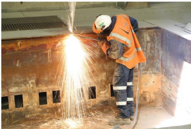
Oxy cutting of pot shells in Line 2 (photo taken 5/2/18)
