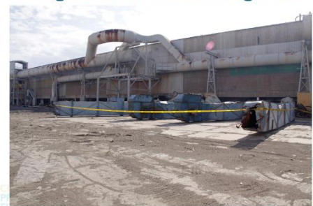
Bucket elevators from L1/2N on hold for asbestos gasket removal (photo taken 25/1/18)
