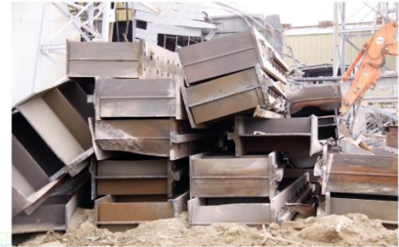
Crane runway beams from Line 3 (each length is 11m long and weighs ~6T)
