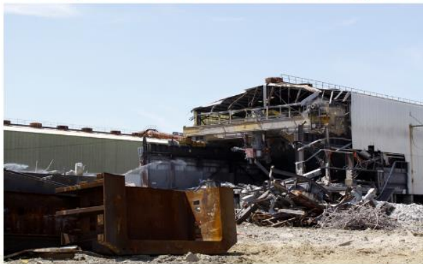
Pot Tending Assembly being pulled out of Line 3 with part of a pot shell in the foreground (photo taken 8/1/18)
