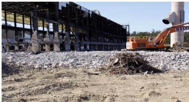
Line 3 South demolition area with concrete stockpile in foreground (photo taken 18/1/18). Concrete is being progressively analysed for contaminants.
