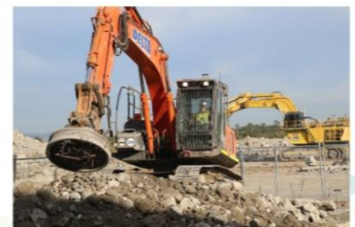
Removal of reo from crushed concrete by electromagnet - May 2018. Concrete to be used for backfill material.
