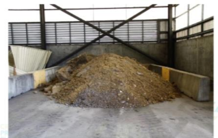
PCB-contaminated soils in 77A awaiting off-site disposal.
