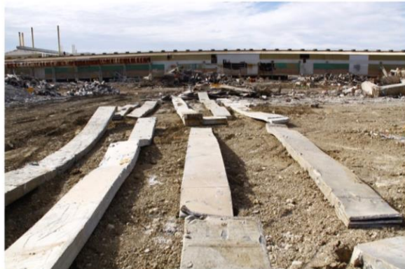
Line 2 and 3 crossover busbar ready to be cut to length and straightened
