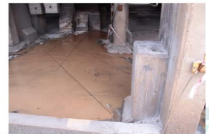
Following saw cutting of Line 1 basement slab
