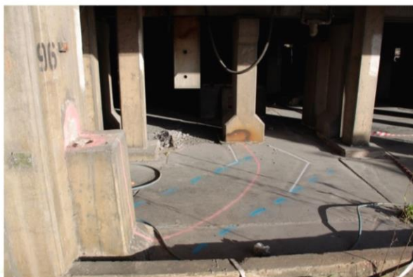
Location and mark out of asbestos conduits in Potline 1
