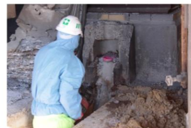
Jack hammering of concrete either side of asbestos conduit by ACM removal crew
