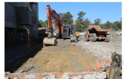
Removal of contaminated/oil stained soils from 3BS substation. Anything with oil staining is checked for PCB's.
