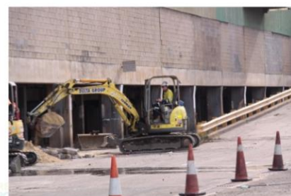
Machine digging of trenches above conduits in Line 1
