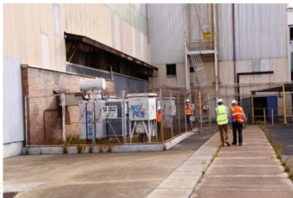
4A north substation at Casting – TL12 transformer footprint had high PCB levels from pre-1985 unit
