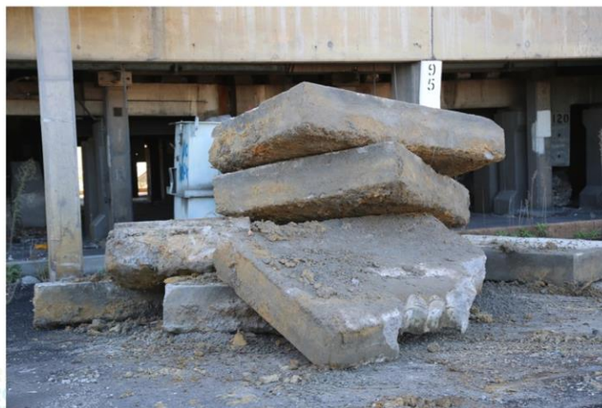
Concrete plinths removed from underneath transformers at 3BS substation. Anything with oil staining will be checked for PCB contamination
