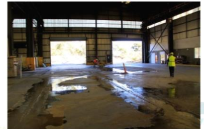
Saw cutting of slab in building 77A (old Remelt facility) to determine content of voids (old melting furnace pit, crucible pit and three scrap bucket pits).
