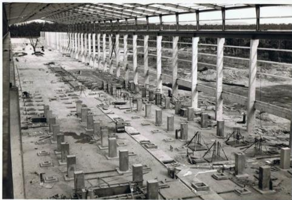
KK-107 26 June 1968 Looking south from Potroom Building 3A crane rail level. Predominant columns are for potshell support. Note pot exhaust trench on centreline of building. Historical photographs from Line 1 construction being used to provide clues on presence of asbestos
