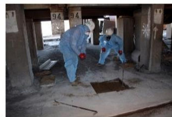
Six locations directly underneath the pots checked for presence of asbestos
