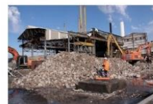
Validation sampling of concrete from the Casthouse (20/7/18). Results show that the concrete is suitable for backfilling.
