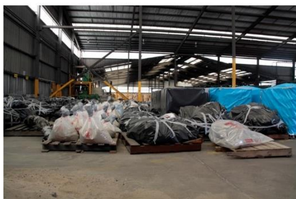
Asbestos conduits and soils wrapped in plastic and stored in Carbon Plant
