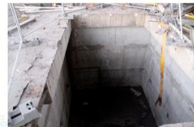
Spacer storage pit following removal of hydraulic cylinder and prior to backfilling with clean concrete.
