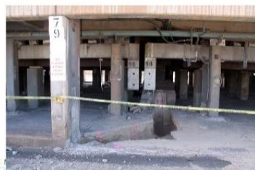
Line 1 conduit trench that has failed validation testing
