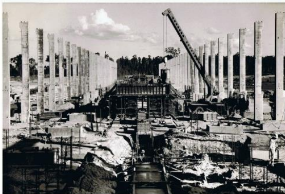
KOT-05 4.8.69 Construction of raised central floor in potroom extension. Exhaust trench in centre foreground. Historical photograph of Line 1 south construction down to Pot 64
