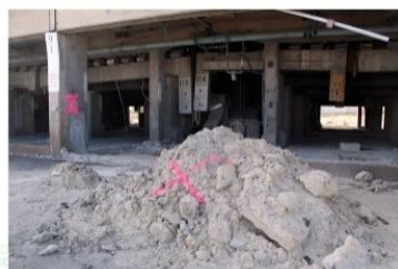
Line 1 soil removed from a conduit trench that has failed validation testing
