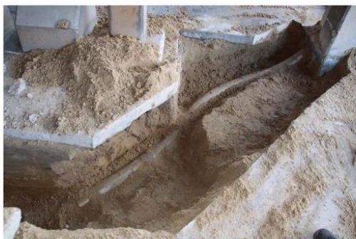
Asbestos conduit in Line 1 following machine and hand digging
