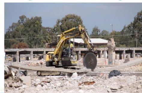
Cutting of busbar using an excavator-mounted saw.
