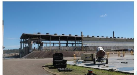
Line 1 Demolition - Long Reach removing alsynite sheeting (photo taken 6/9/18)
