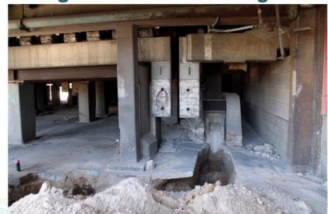
Removal of Line 1 asbestos conduits complete (13/9/18) All trenches validated to be free of asbestos as @ 12/10/18
