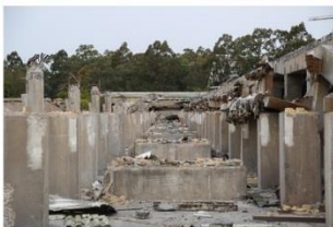
Line 1 pot superstructure column foundations
