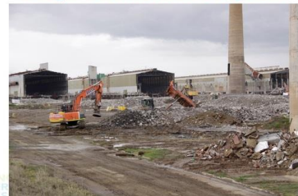
Line 1 concrete - transported to SW corner for sorting. Magnetic separation to remove reo - 11/10/18.
