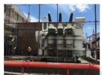
Jacking & skating a Line 1 transformer - 10/12/18
