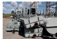
Removed radiators & conservators - 15/11/18
