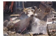
Compressor House (57C) Foundation Removal - 20/10/18
