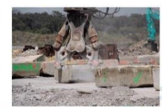
Cracking of clean concrete foundations
