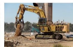
Removal of Line 3 North Scrubber Fan Foundation 15/11/18
