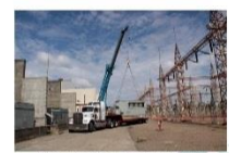
Removal of a Line 2 rectifier cabinet - 27/11/18
