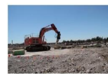
Cracking of clean concrete foundations
