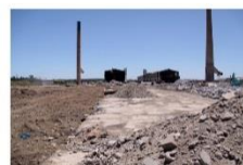
Piles of sieved concrete material from foundation footprints
