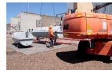
Removal of oil conservators in Switchyard photo taken 12/11/18
