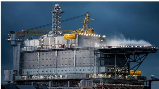
> *Figure 3-3 Aluminium living quarter structure from Leirvik AS, size 92 m x 28 m x 30 m (total of 1500 tons aluminium material)*
