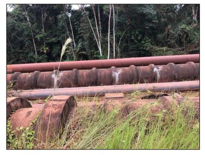
Figure 4.15 Example of small repairs of concrete pipes
