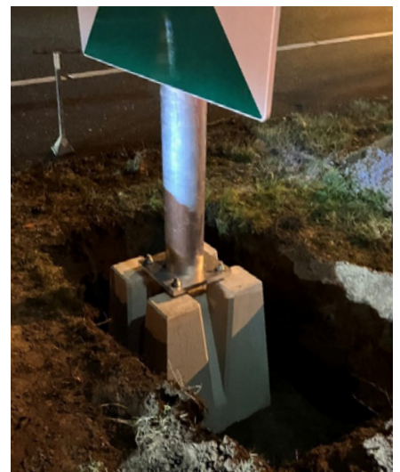
Prefabricated foundation for quick installation
