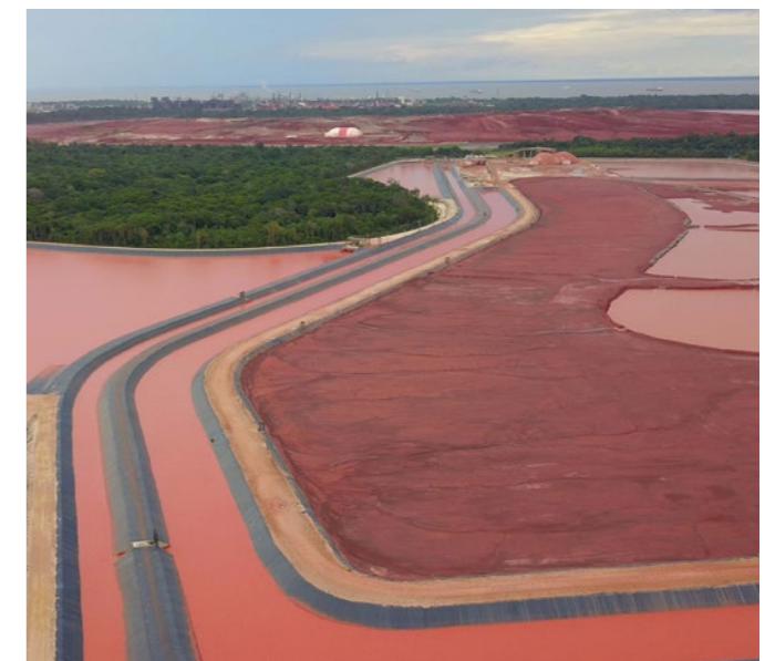
Bauxite residue disposal area at Hydro Alunorte, Brazil.
